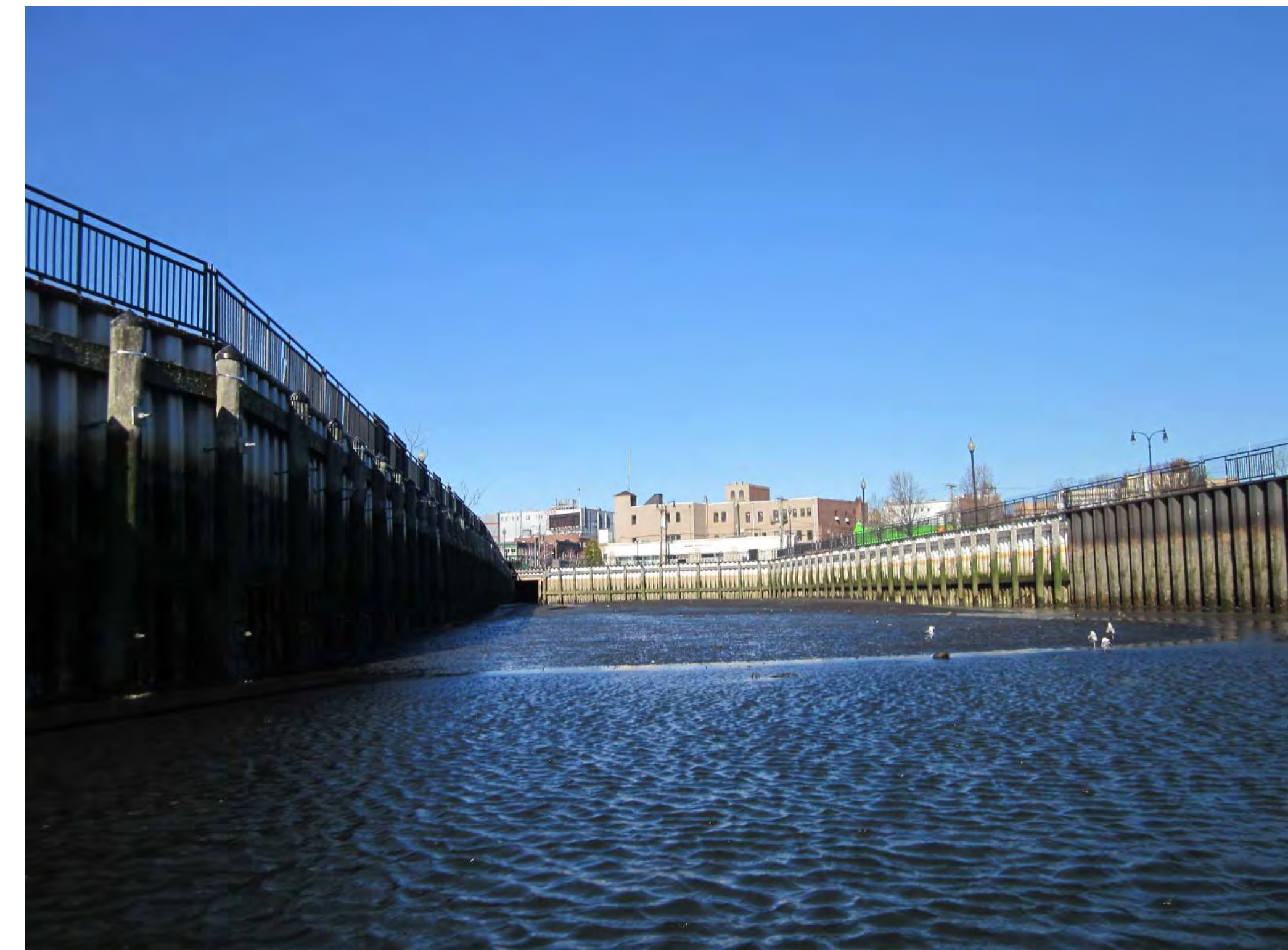
General View of Cove- Looking West
