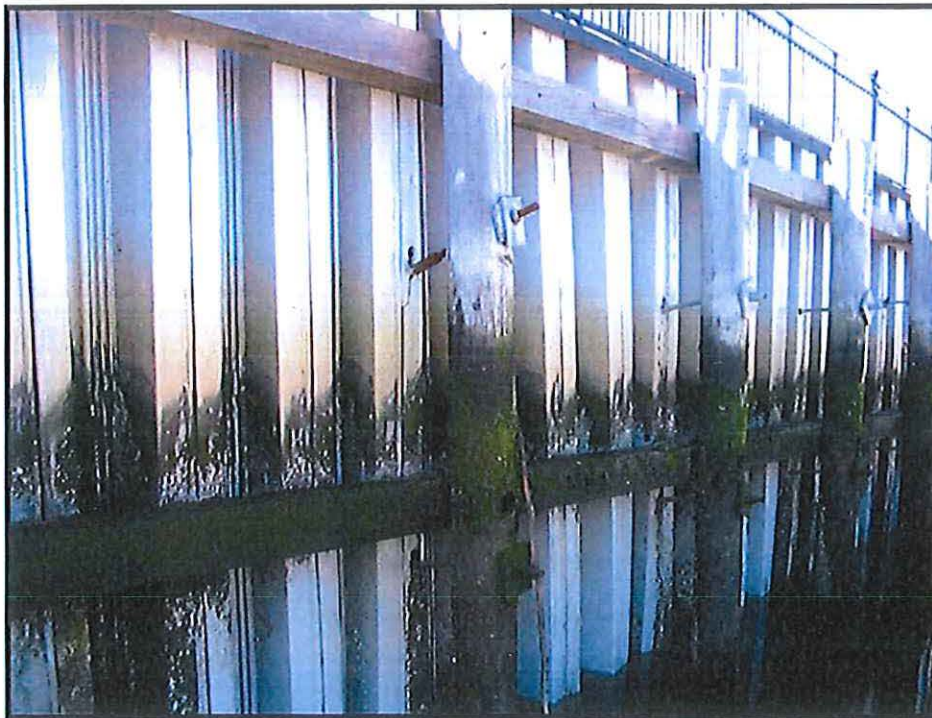
Photo No. 12 – Not crack in the sheet piling at tie-rod location due to settlement. This detail was not provided on the Contract Drawings.
