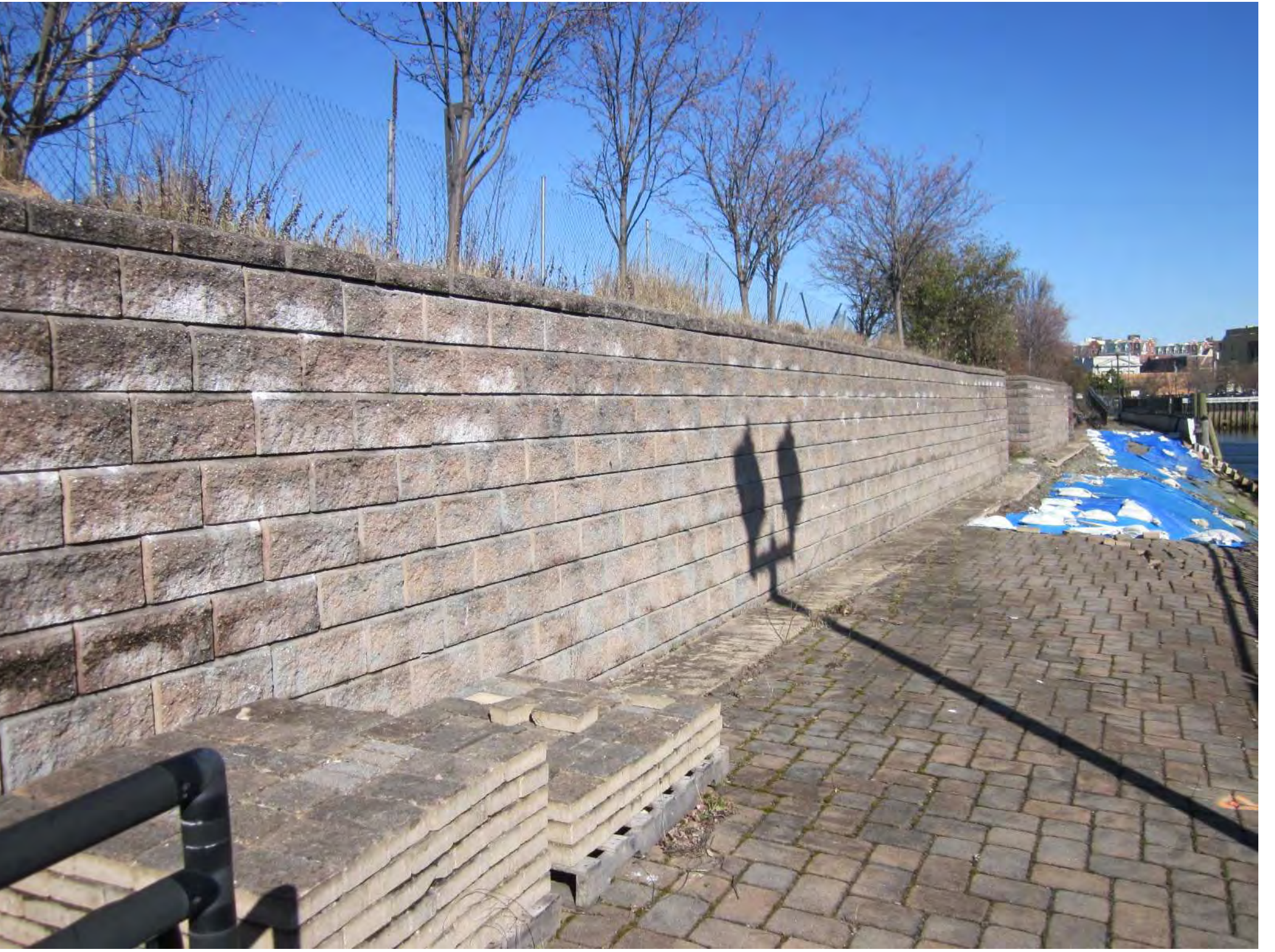
Walkway Section 2 - Looking North
