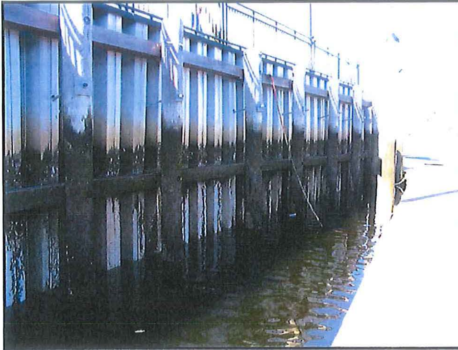
Photo No. 1 – The replacement vinyl sheet pile bulkhead.
