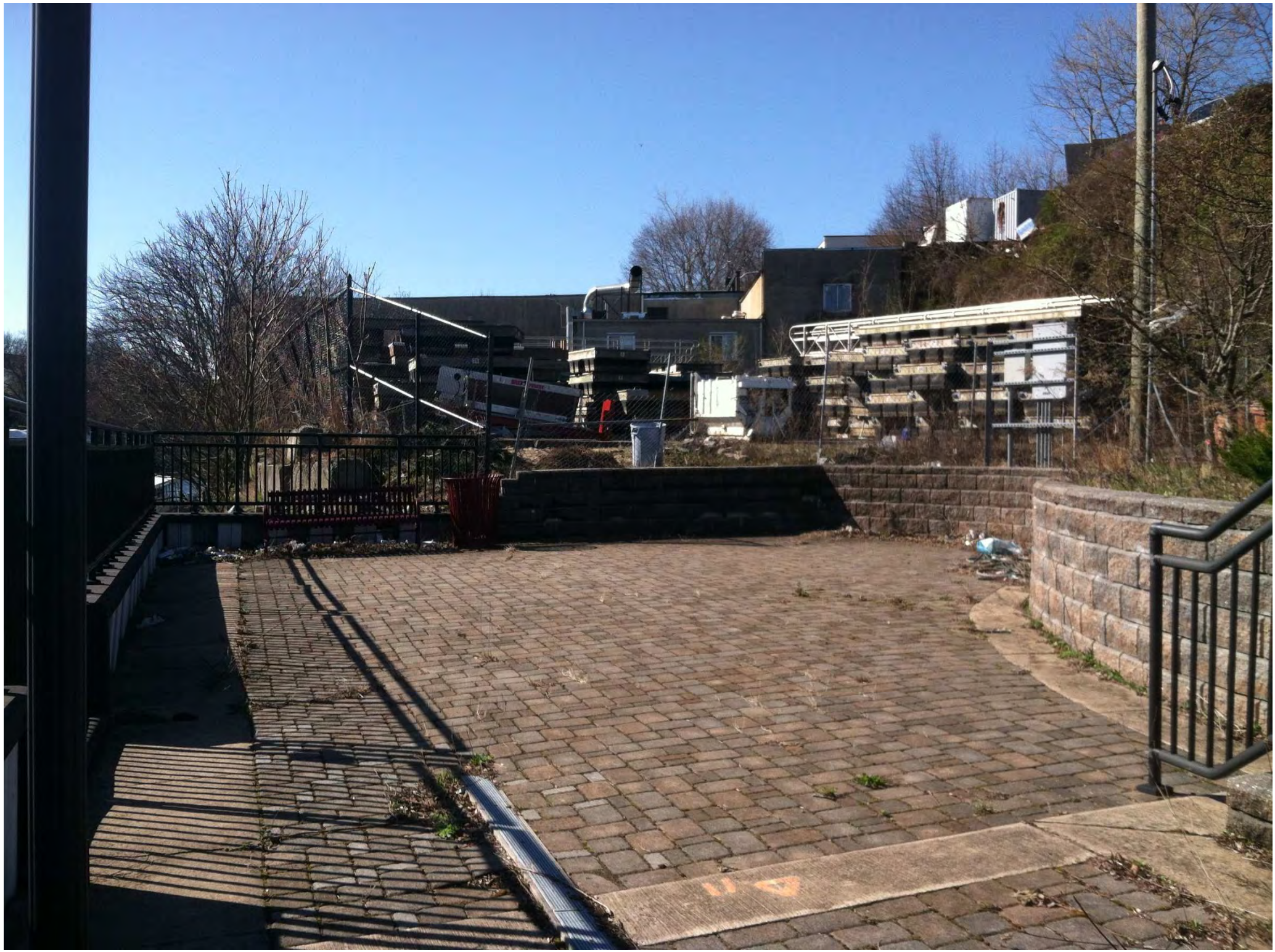
Walkway South End- Looking South
