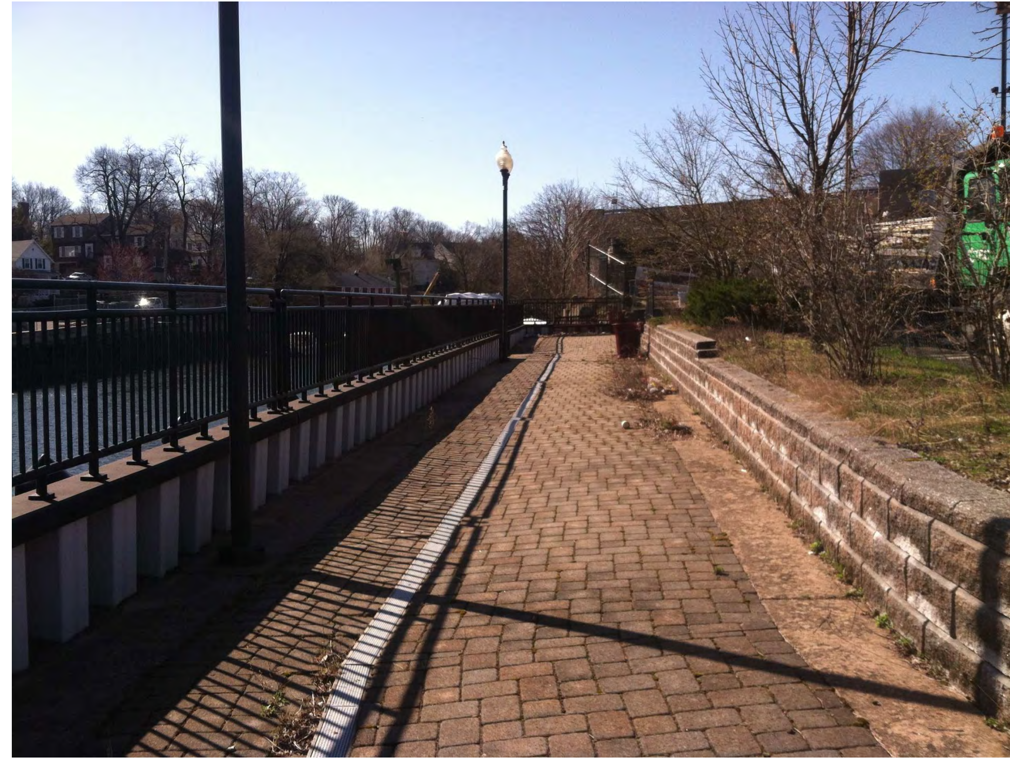
Walkway Section 1 - Looking South
